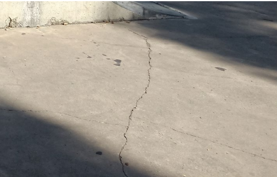
Concrete surface is deteriorated causing safety hazard. Poor surface limits functionality to skateboard wheels.
