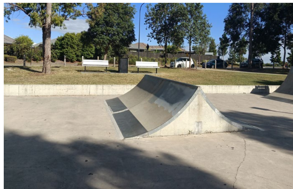
Existing slabs has surface cracking, degraded concrete edges and corners, uneven, open and degraded expansion joints.
