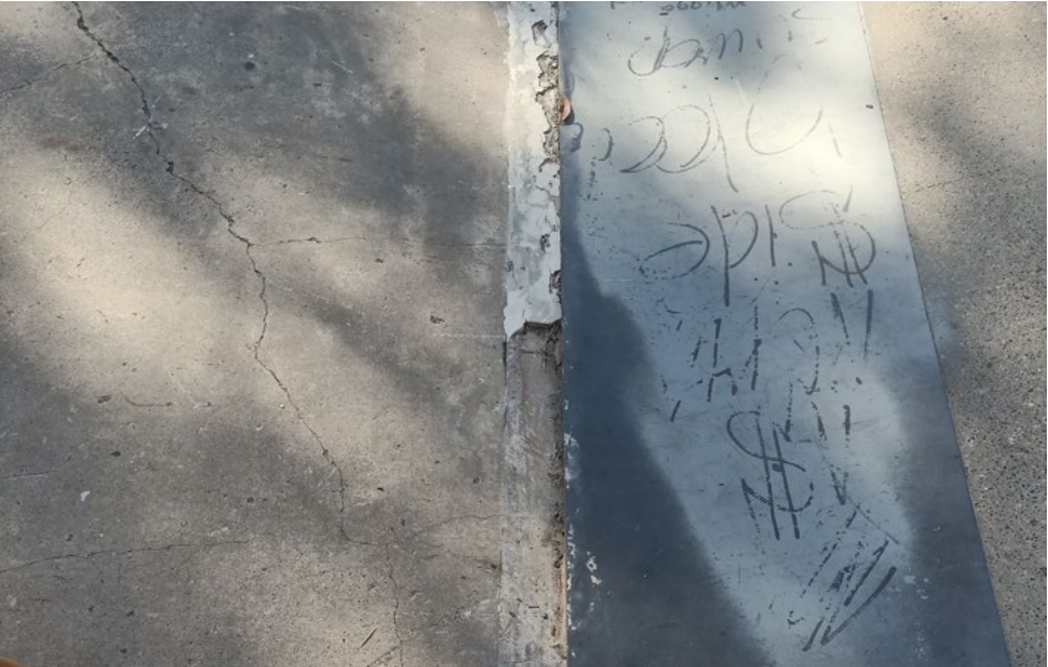
Significant uneven, open and degraded expansion joint. Creates major safety hazard and on going maintenance.
